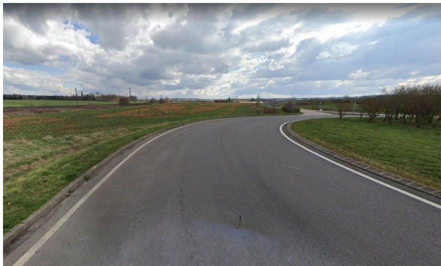
Figure 27 : Photographie issue de Google Street View – D590 – Moncel-lès-Lunéville
